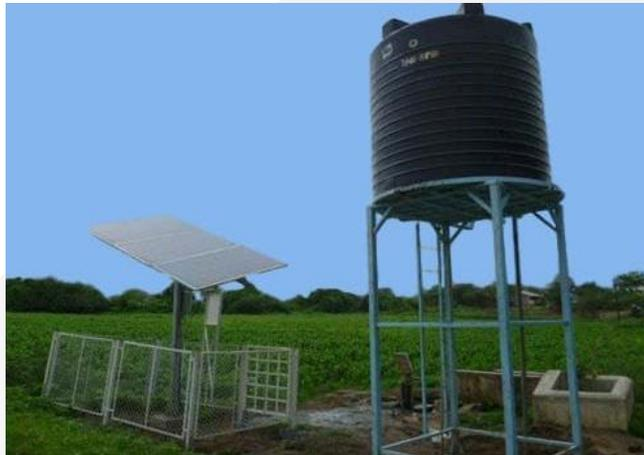
Well pumping with elevated storage tank
