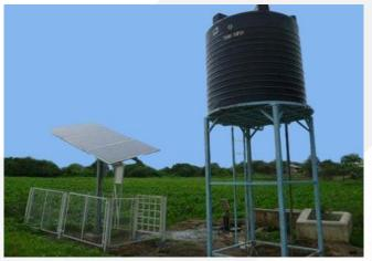
Well pumping with elevated storage tank
